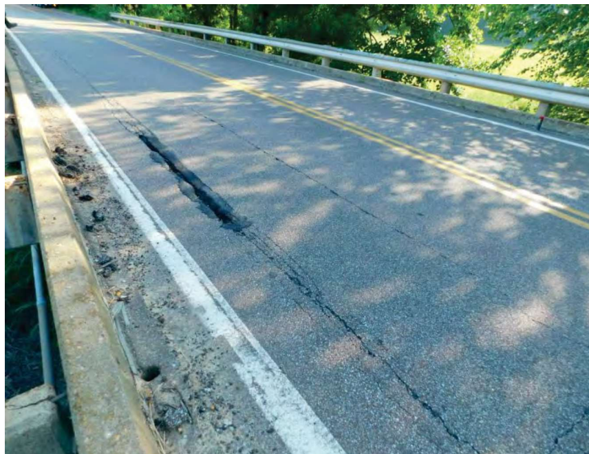
VIEW ACROSS TOP OF DECK
