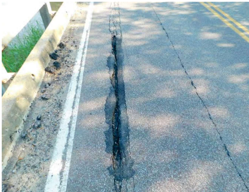
SPAN 1 POT HOLE
